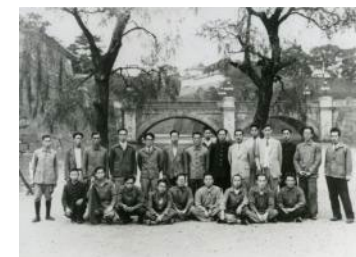
Oku-Goten in imperial palace completion ceremony
