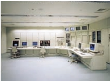
Fire Monitoring Panels in Control Center
