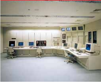
Fire Monitoring Panels in Control Center
