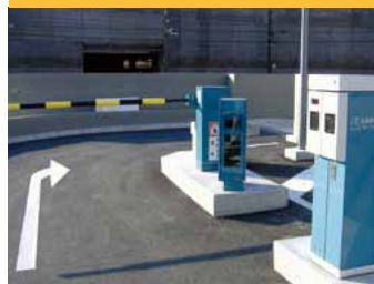
Parking Control System
