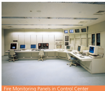
Fire Monitoring Panels in Control Center
