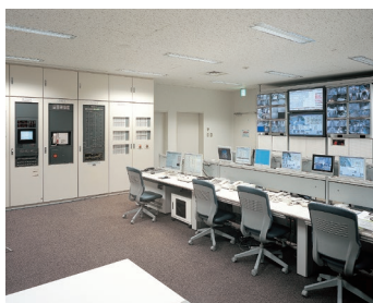
Fire Monitoring Panels in Control Center
