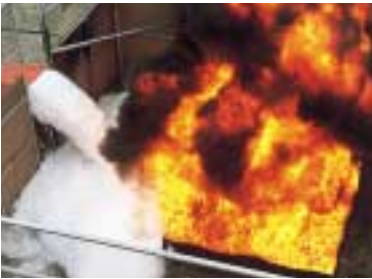
High-Expansion Foam Extinguishing System
