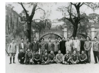
Oku-Goten in imperial palace completion ceremony
