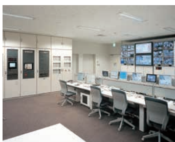
Fire Monitoring Panels in Control Center
