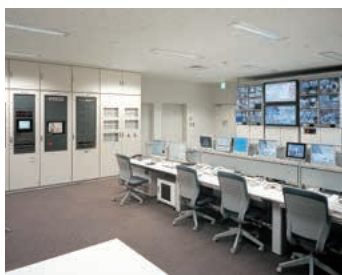
Fire Monitoring Panels in Control Center
