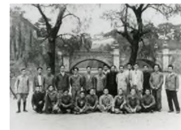
Oku-Goten in imperial palace completion ceremony
